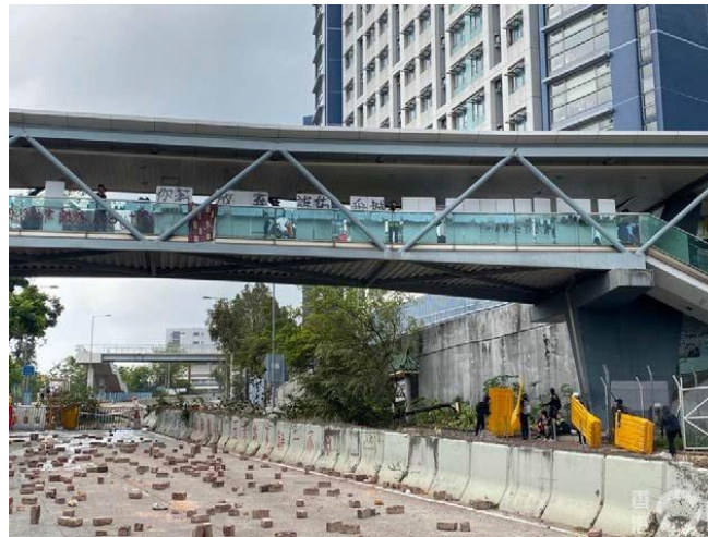
Image 4-107: Cornwall Street outside residential halls of CityU was blocked (Image source: HK01)
